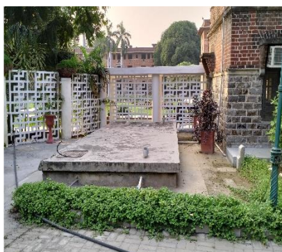
Rain water storage tank
